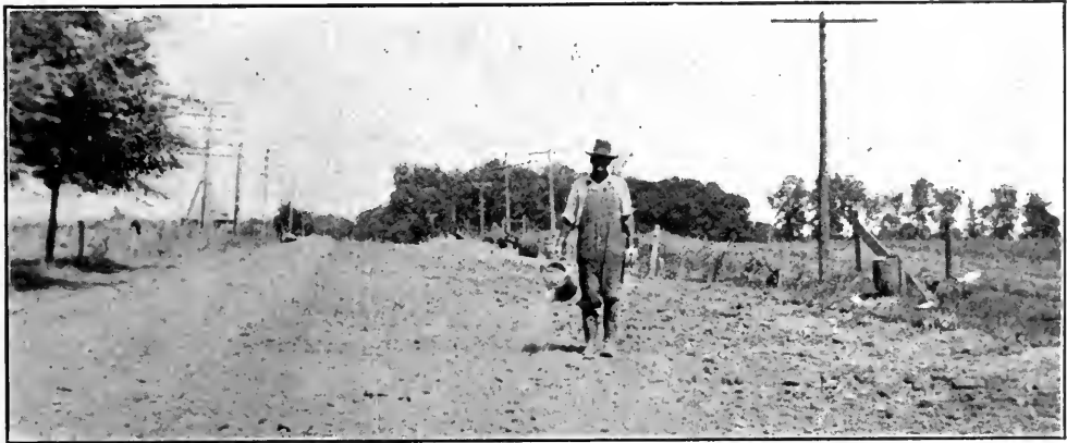
A PORTION OF ROUTE 5, ILLINOIS STATE HIGHWAY, BUILT BY McCALL CONSTRUCTION COMPANY, USING CALCIUM CHLORIDE FOR CURING
